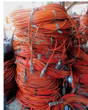
Damaged cables awaiting repairs.
